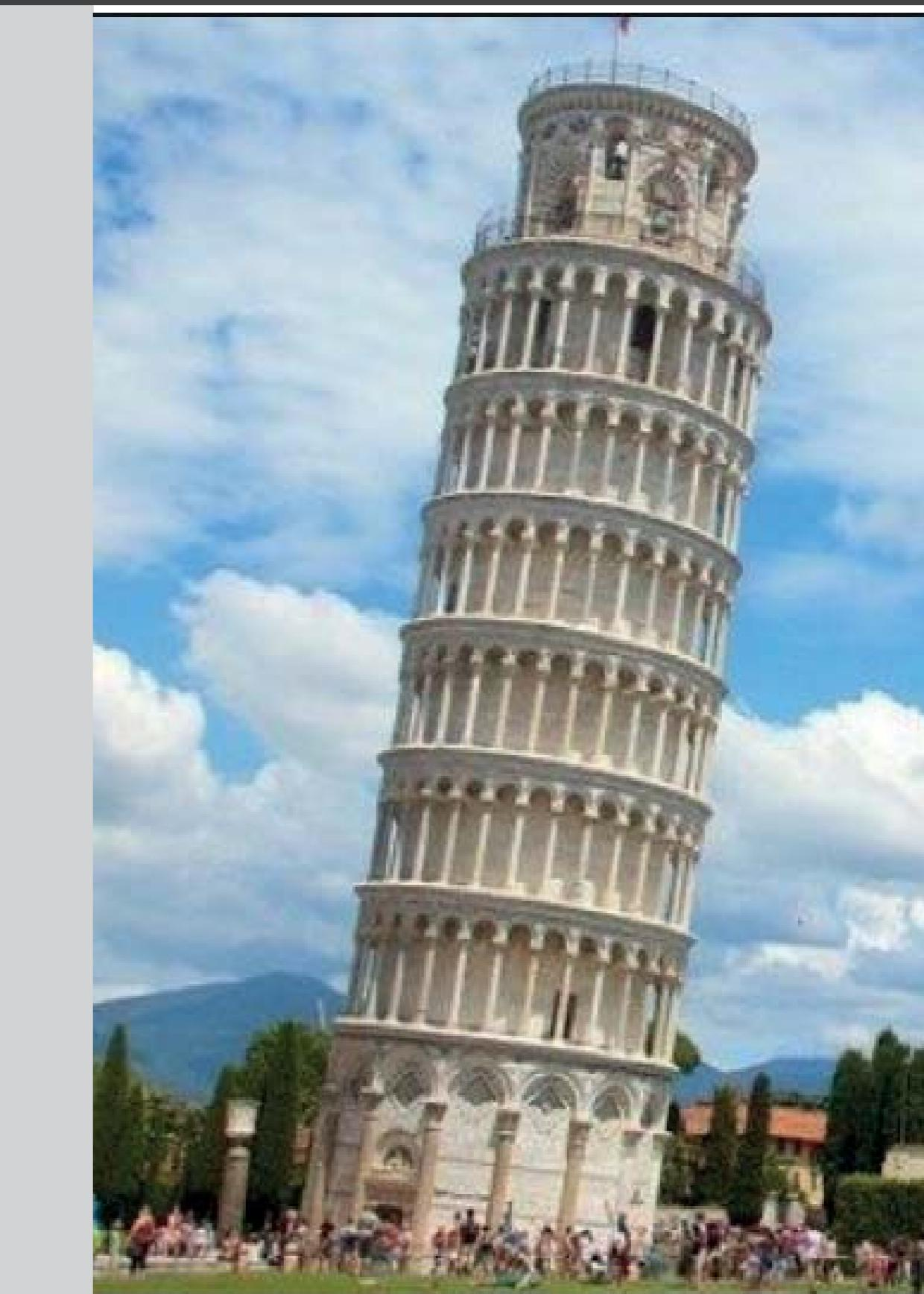
**Examples of geotechnical challenges associated with sandy soil:** (Left) Differential settlements of the Pisa tower in Italy. (Below) landslide problematic and internal erosion in sands.
